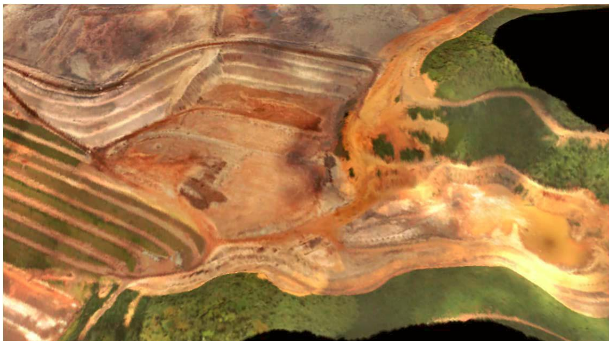
Figura 9 - Fundão Dam in January, 2014 showing left abutment setback and adjacent Grota da Vale (Disponível em: < http://fundaoinvestigation.com/the-report/ >. Acesso em: 18 ago. 2020.)
